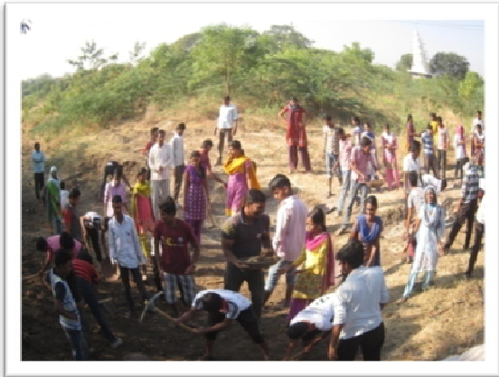
Expansion of Percolation Tank
